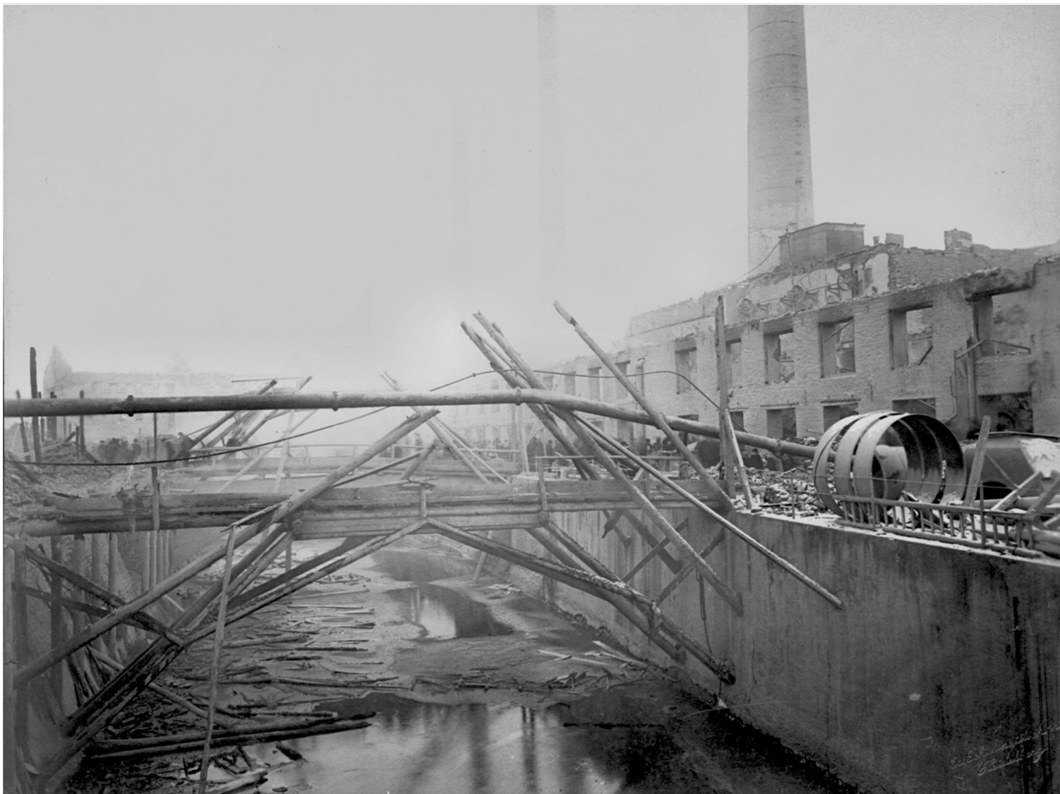
Cement mill building at the millrace AFTER THE FIRE of February 4, 1895.
