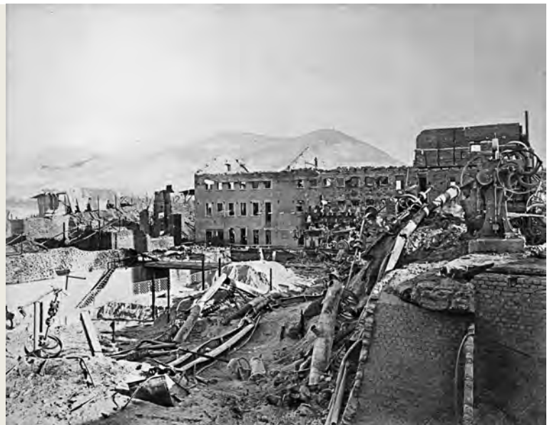
RAW MILL BUILDING after the fire, February 1895.
